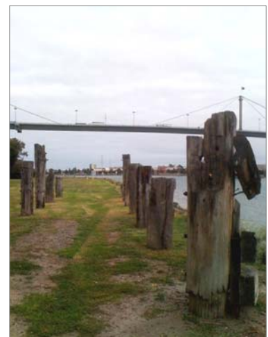
Historic timber wharf piles at Fishermans Bend
